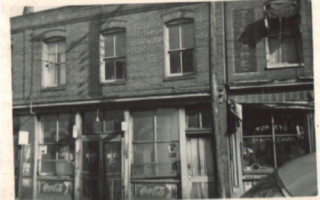
Figure 1. 411 Brook Road, approximately 1955, City of Richmond Assessors Office. Some original components/materials of the storefront are present.
