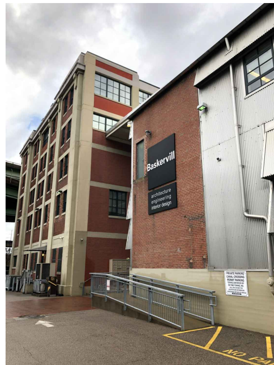
2 Existing Building - Drive Aisle
