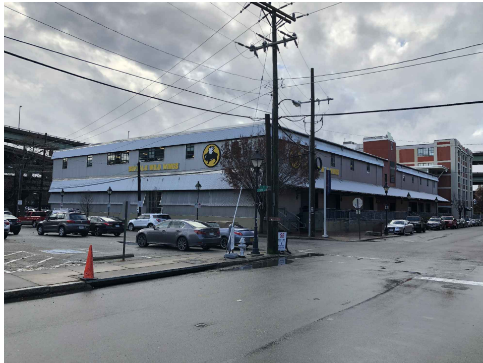
6 Existing Building - East Carry Street and 15th Avenue
