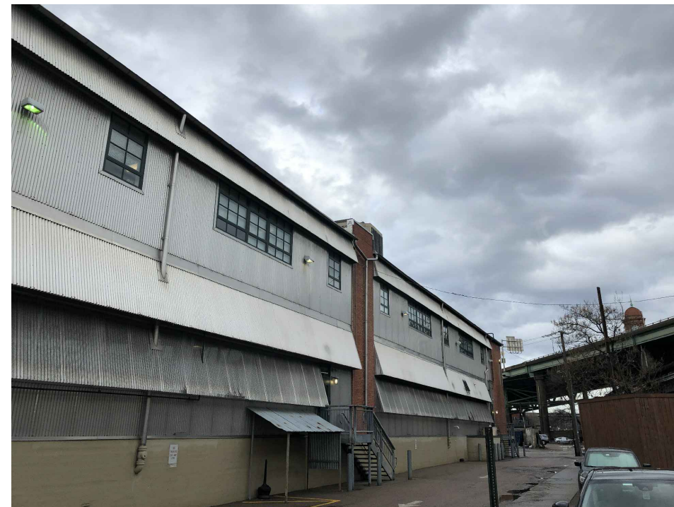
1 Existing Building - Drive Aisle
