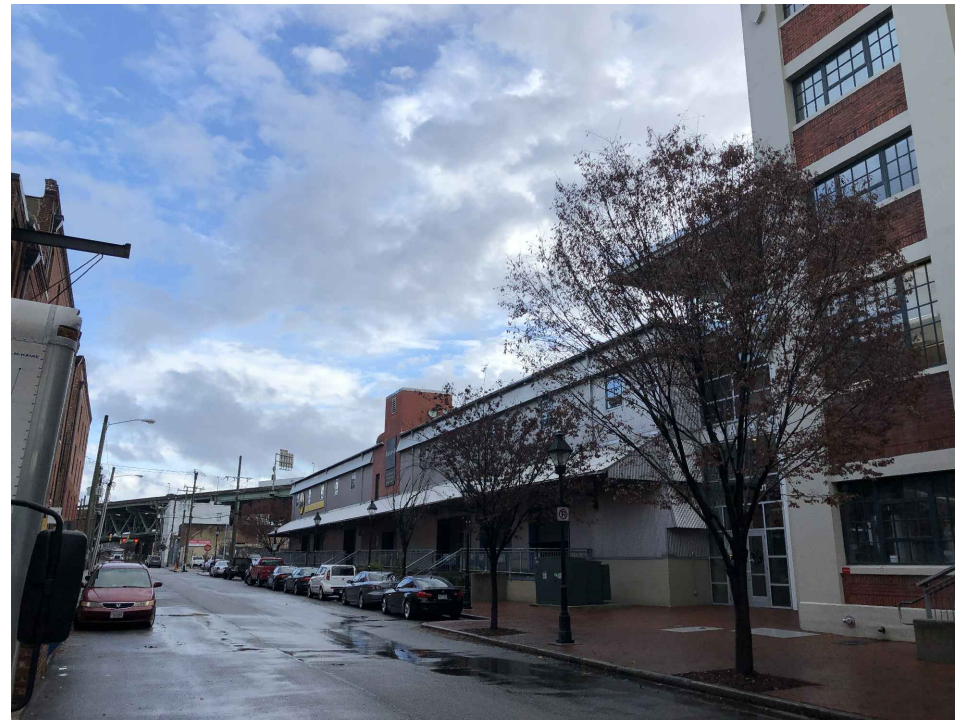
5 Existing Building - 15th Avenue
