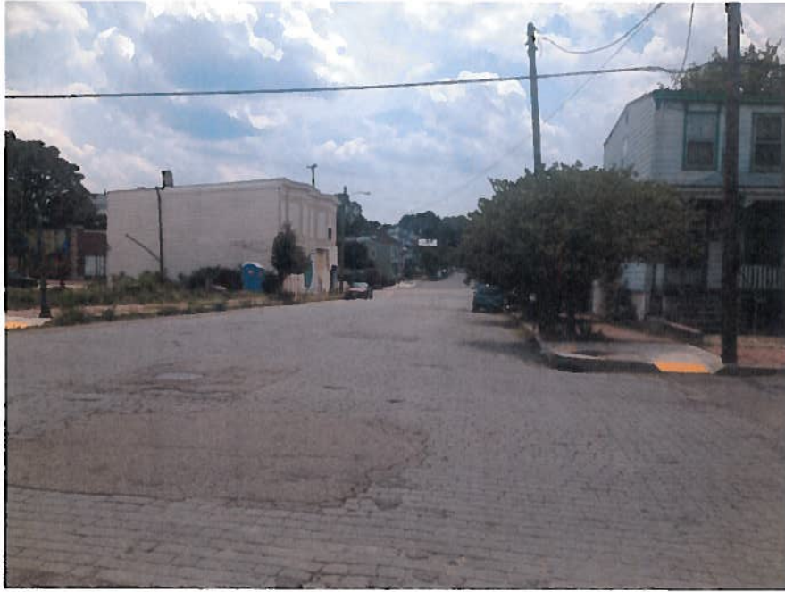
View South on 24 th Street
