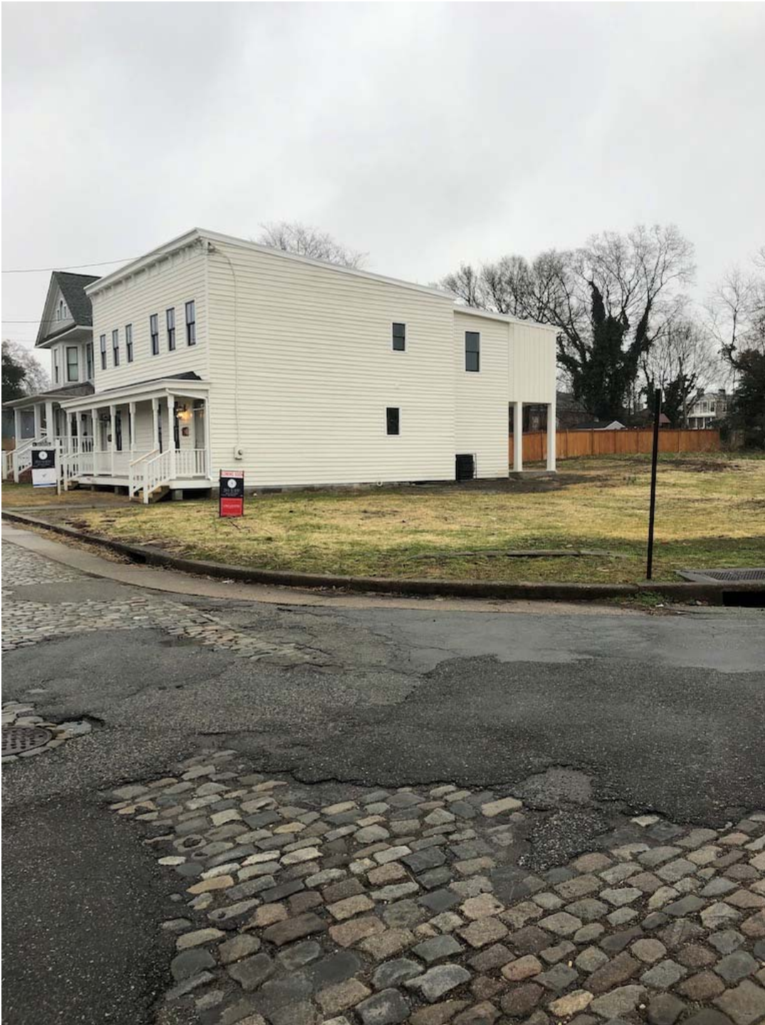
2311 Carrington view looking East
