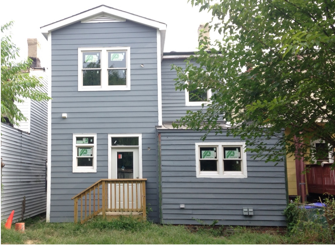
South Elevation – August 2017
