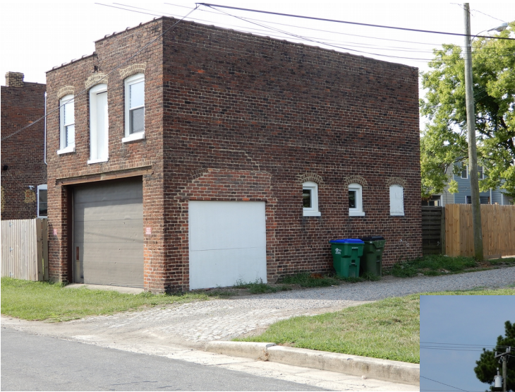
High Half-windows facing Alley (left & below)
