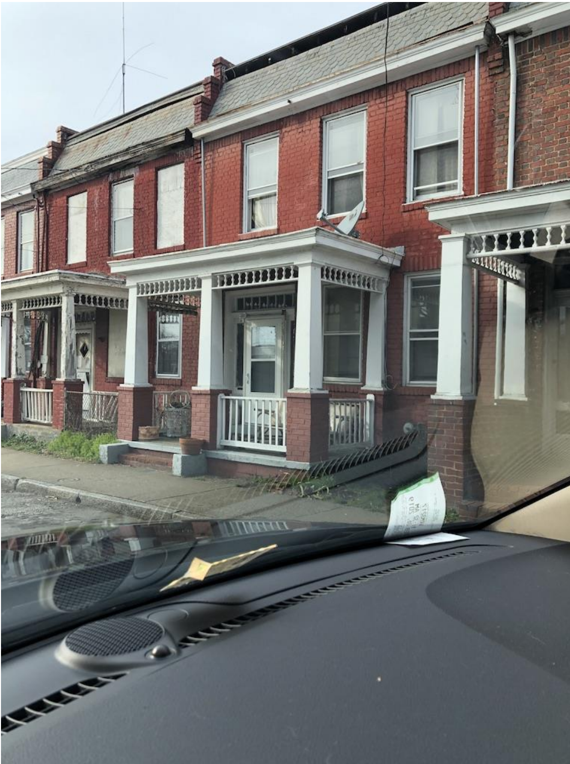
Front Elevation Barton St. with similar "false mansard" roof.
