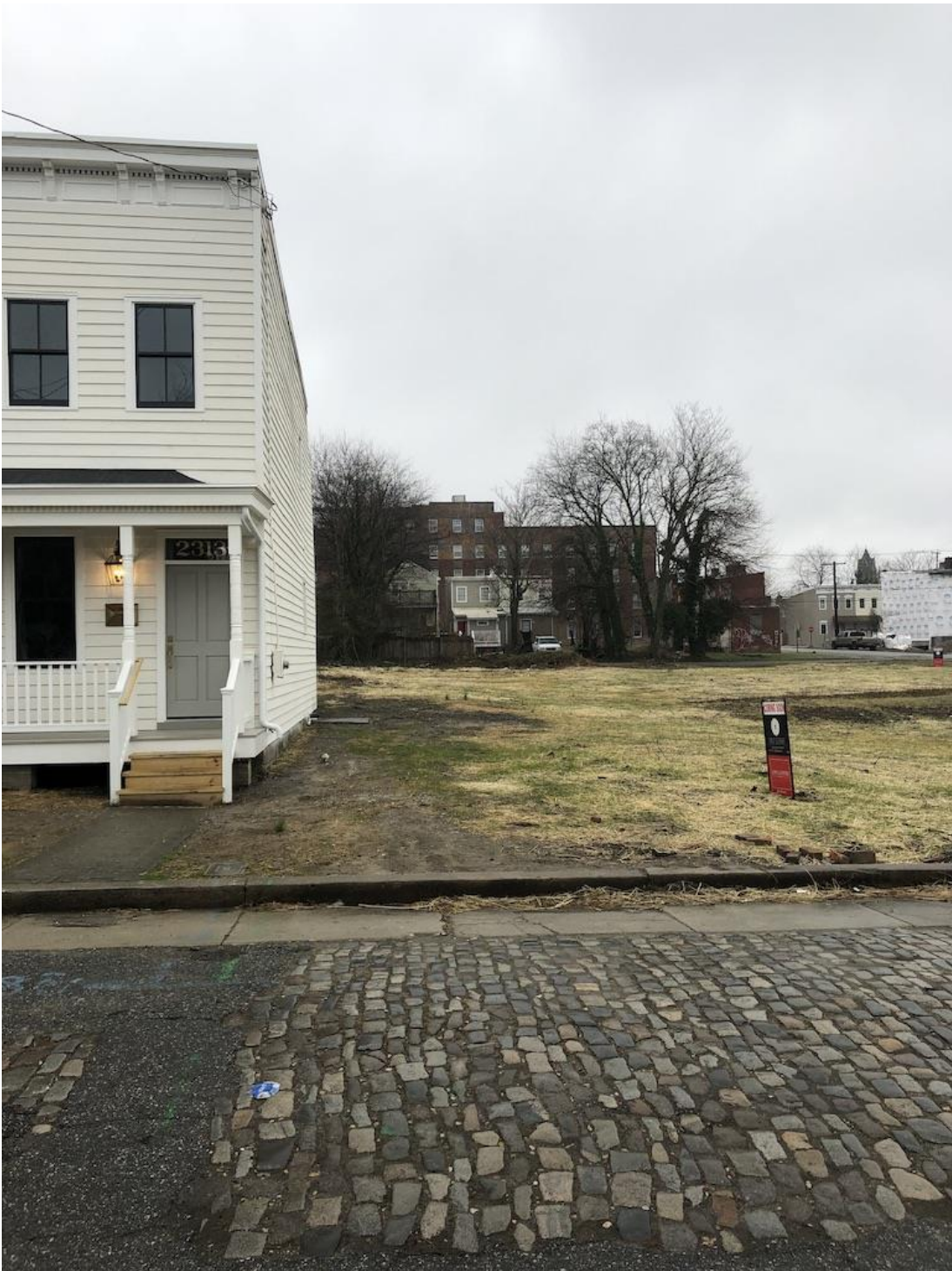
View of 2311 from street
