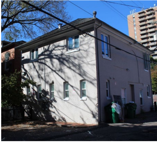
Figure 3. Example of outbuilding on W. Franklin St.
