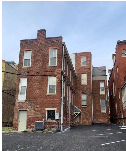
Figure 2. Rear façade, view from rear alley
