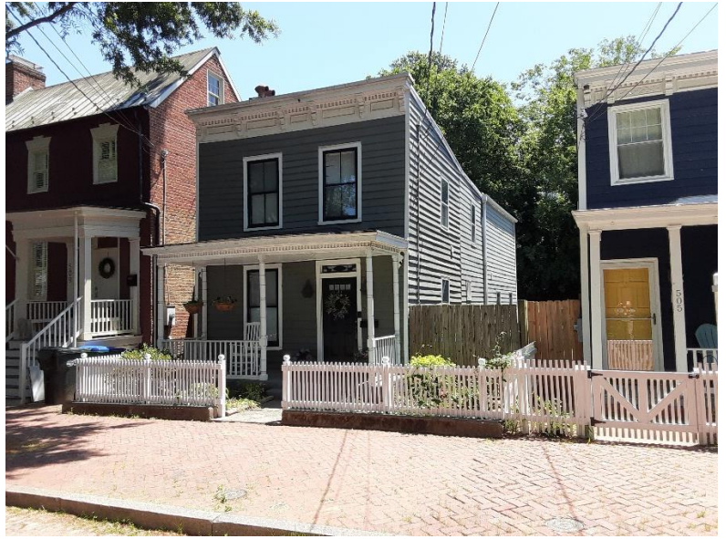
Figure 2. 507 N. 27th Street, view to location of the sunroom and terrace.
