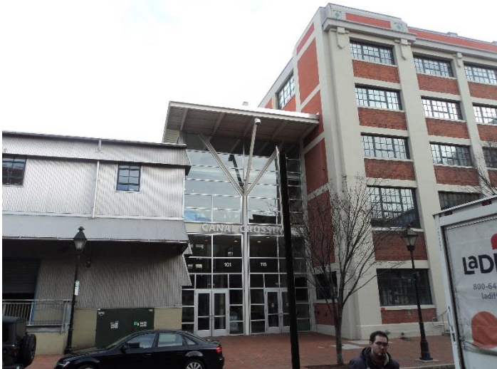
Figure 3. 101 South 15th Street, existing entrance.
