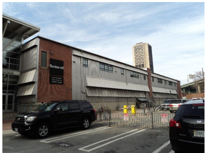
Figure 4. 101 South 15th Street, side elevation.
