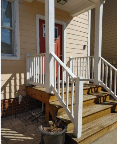
Figure 3. Existing back porch with wood railings
