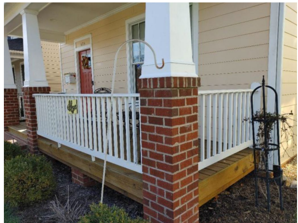
Figure 2. Existing front porch with wood railings
