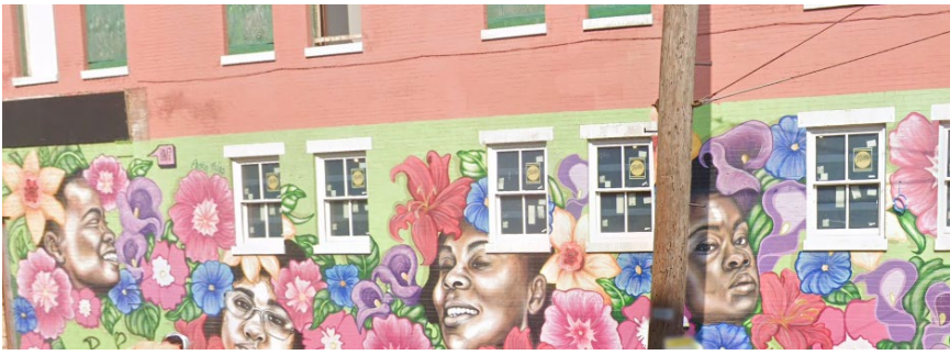
Figure 8. Example of CAR approved mural where stone lintels were not authorized to be painted.
