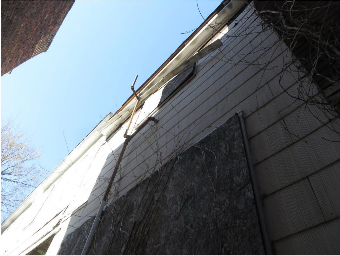
Photo 5: East elevation, view of the asphalt siding at the northern end
