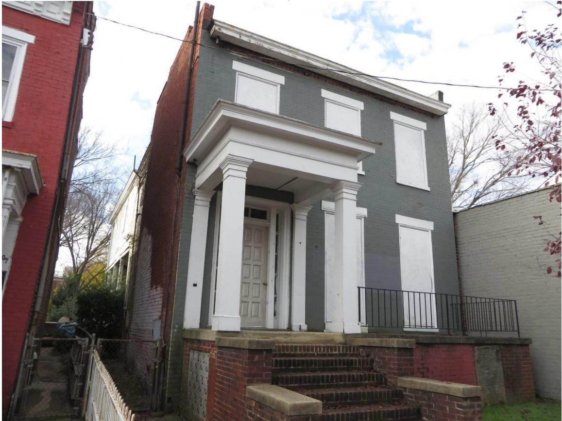
Photo 2: North and east elevation, view to the northwest
