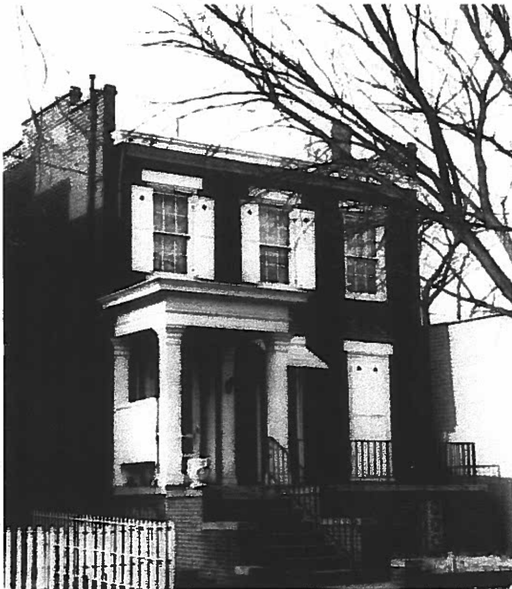
Photo 1: North elevation, historic photo showing wood shutters
