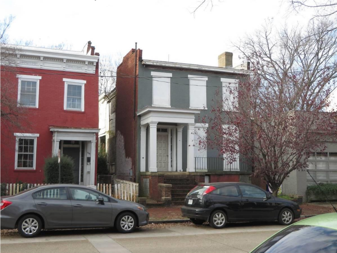
Photo 1: North elevation, view to the southwest
