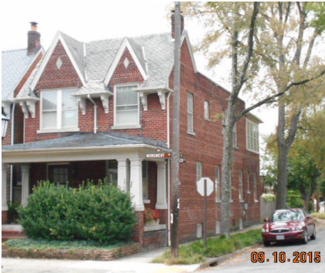
Figure 3. 3225 Monument, view of storm windows on front and side elevations. 2015, City Assessor's Image.
