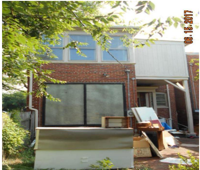
Figure 4. 3225 Monument, view of storm windows on rear elevation. 2017, City Assessor's Image.
