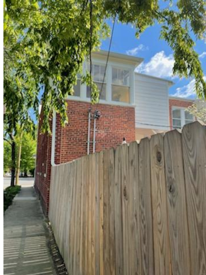
Figure 2. 3225 Monument, rear elevation from Tilden Street
