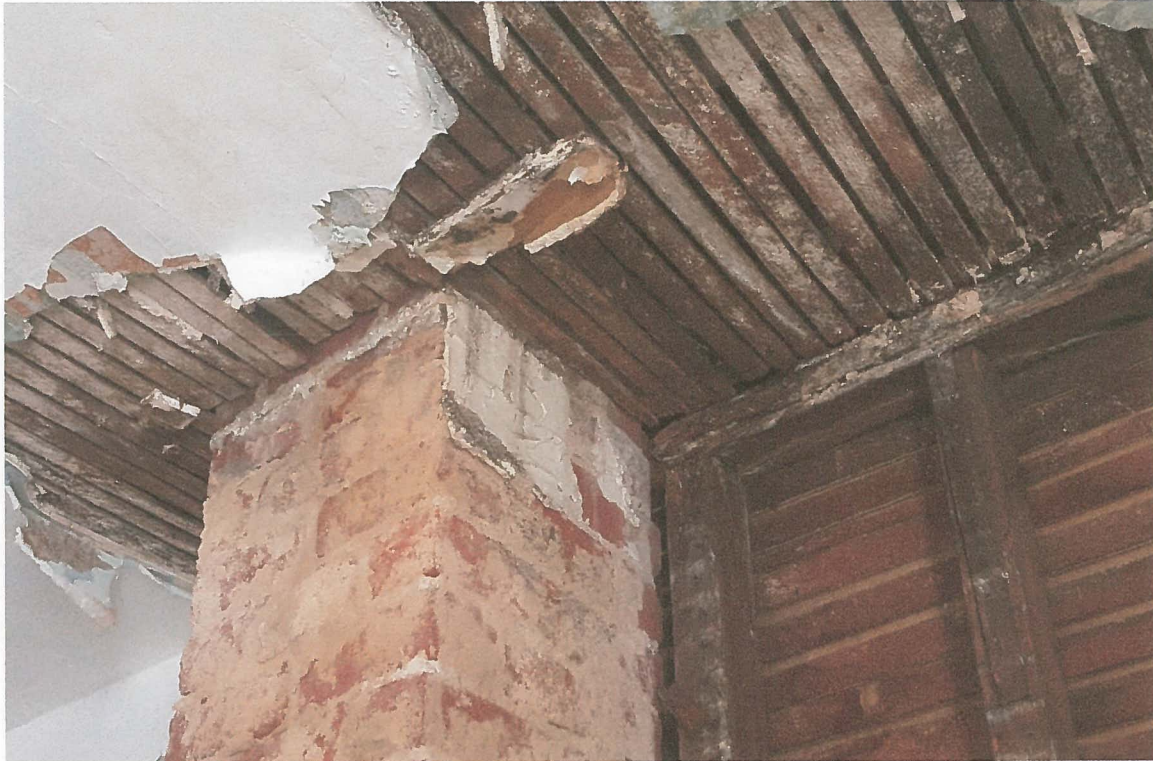
Photo 8. Water damage to plaster ceiling in Foyer on 1 st Floor due to leak above
