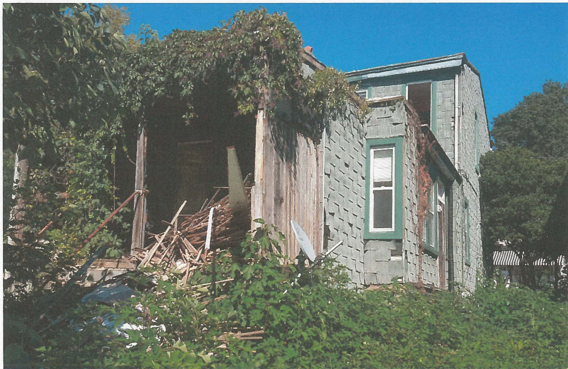
Photo 2. Rear Elevation with collapsing porch at left, North Elevation at right
