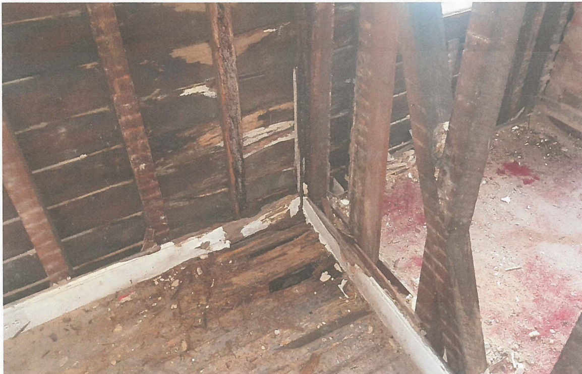
Photo 6. Exterior stud wall along the Southern elevation and floor in Living Room rotted due to water damage; sill and joist damage below flooring
