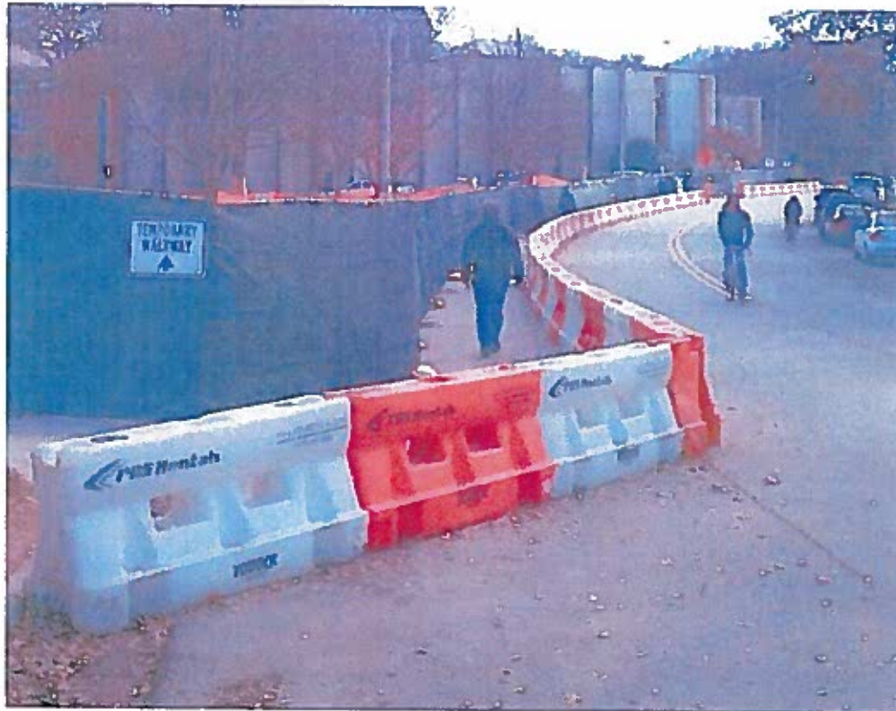
Example of protected temporary sidewalk.
