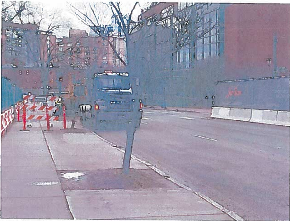
Sidewalks on both sides of street closed in Richmond
