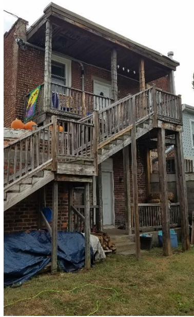
Figure 6. 3105 East Marshall Street, rear elevation.
