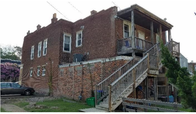
Figure 5. 3105 East Marshall Street west and rear elevations.
