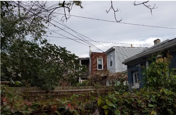
Figure 7. 3105 East Marshall Street, side and rear elevation.
