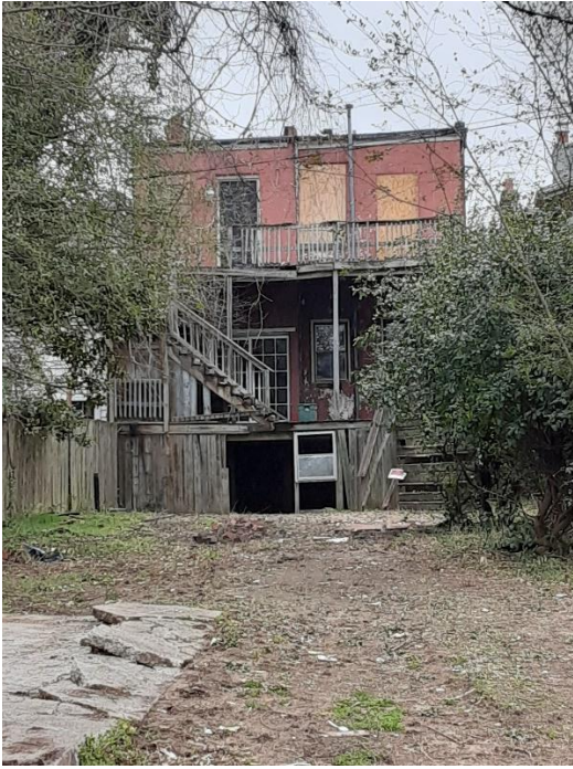
Figure 5. 2909 E. Broad Street, rear elevation.
