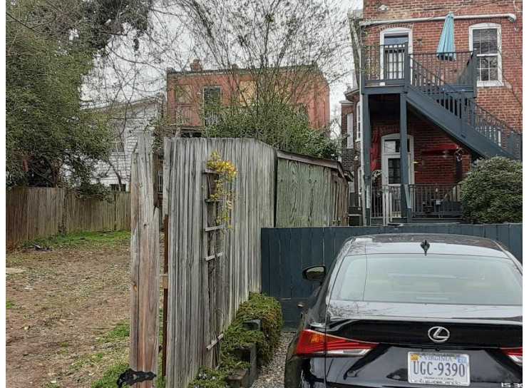
Figure 6. 2909 E. Broad Street, rear elevation and neighboring building.
