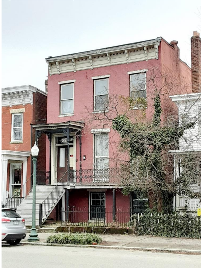
Figure 3. 2909 E. Facade Street, facade.
