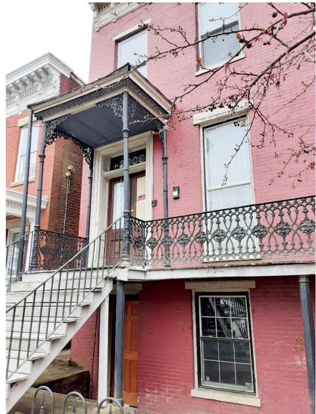
Figure 4. 2909 E. Broad Street, porch and door details.
