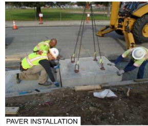
PAVER INSTALLATION
