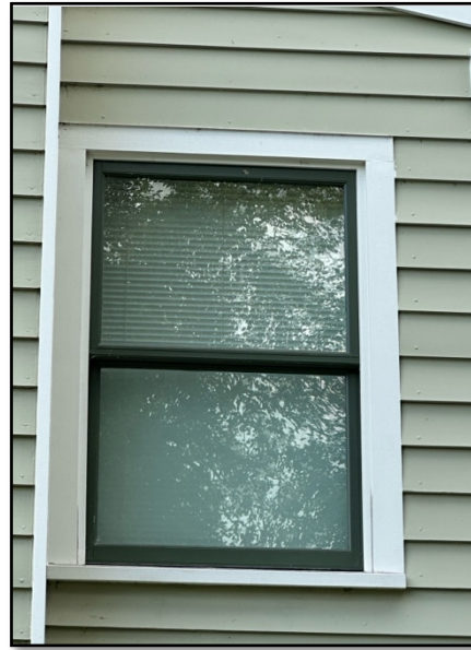
Existing Window on Main Dwelling
