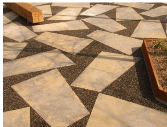
Reclaimed Stone and Porous Paving
