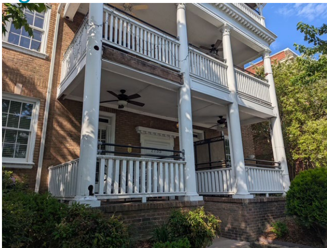
Figure 1. Existing Conditions, facade, April 2026.
