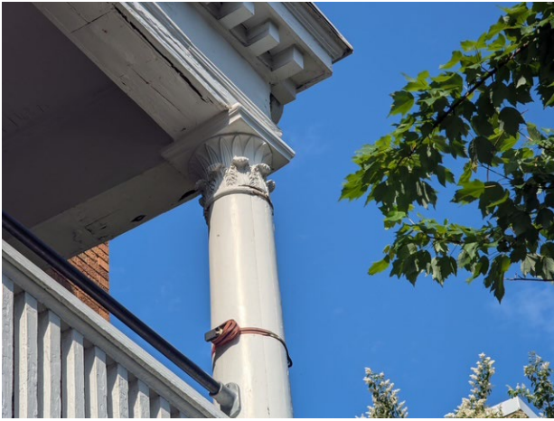
Figure 3. Existing condition of western column. April 2026.
