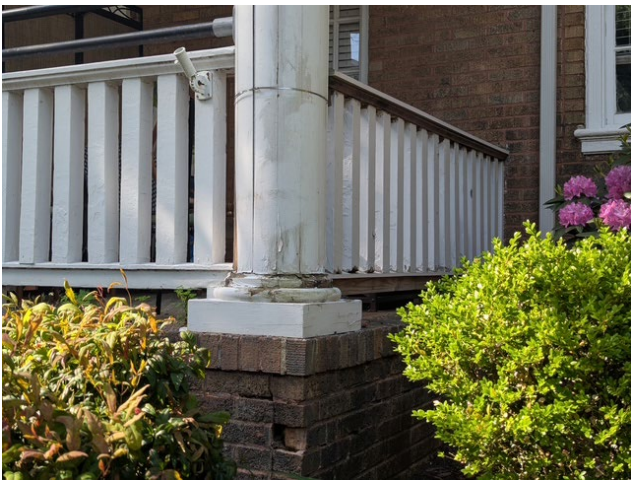
Figure 5. Existing condition of western column. April 2026.
