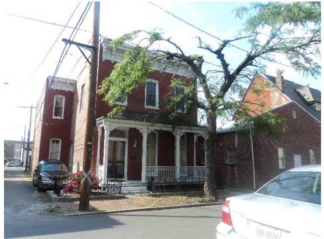
Figure 4. 500 block St. James St, even side
