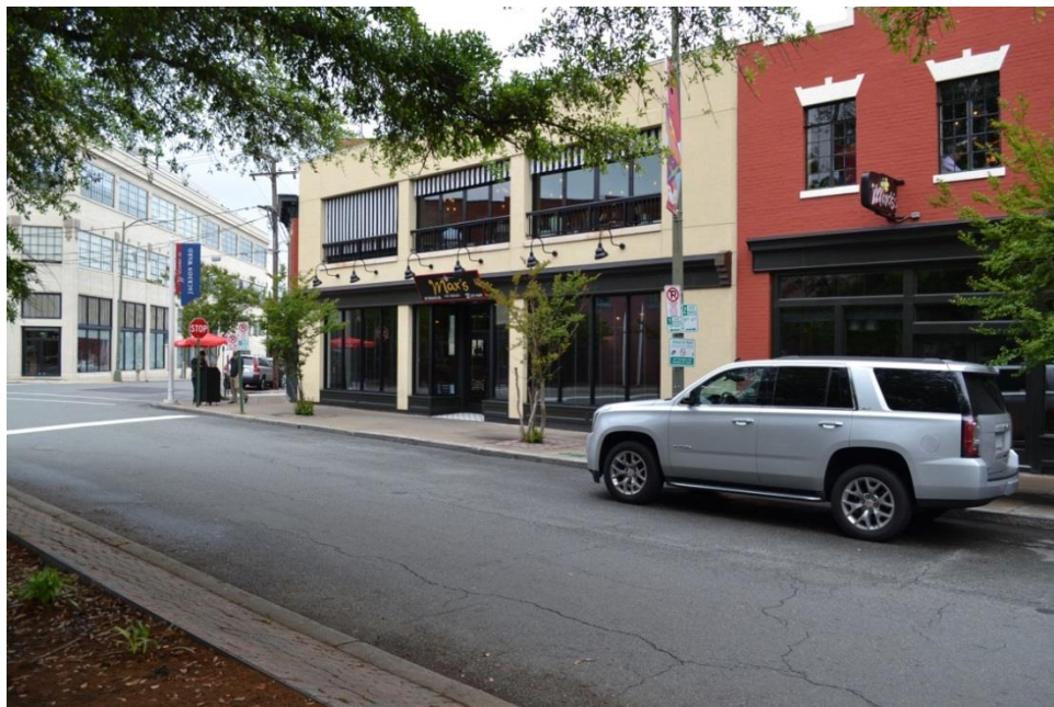
View northeast of 303 and 307 Brook Road that face the plaza. (Source: Liz Sargent, May 2016)
