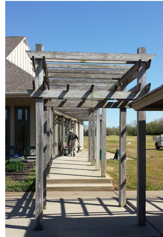
Trellis to be demolished
