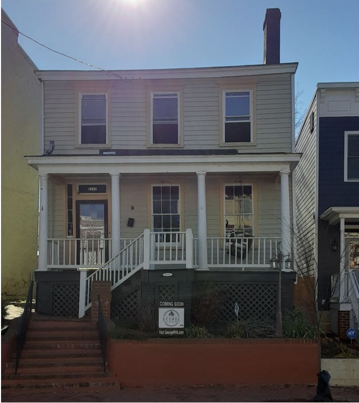
Figure 1. 2115 Cedar Street, facade
