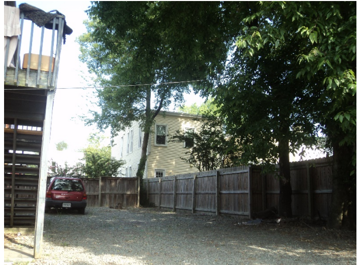
Figure 2. View of rear elevation from alley.
