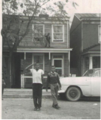
Figure 1. Previous dwelling at 974 Pink Street. Demolished 2001. Image: City of Richmond's Assessor's Office approx. 1955.
