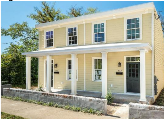
Figure 3. Rehabilitated 970-972 Pink Street.
