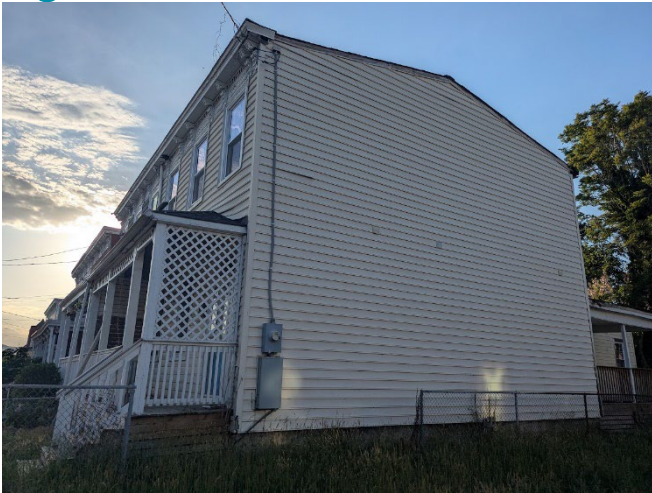
Figure 1: site elevation of the attached buildings at 2222 Venable, showing similar roof form as the proposal
