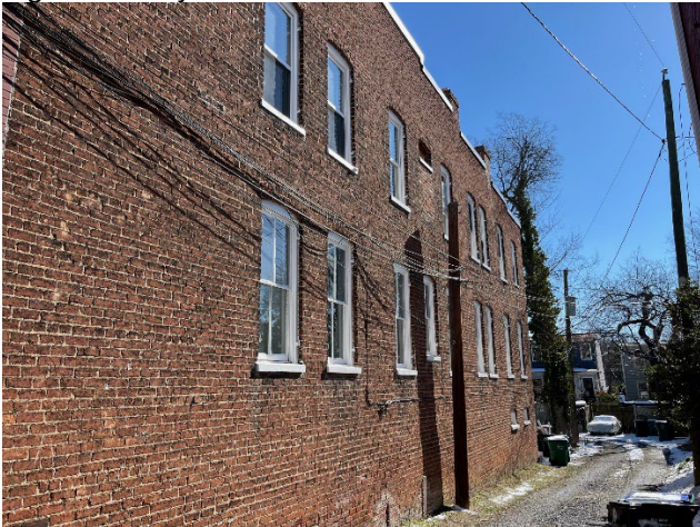
Figure 3. Alley Elevation with infilled window.
