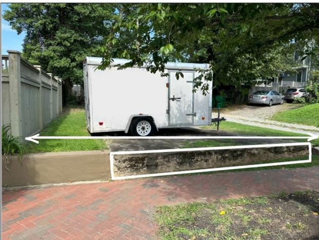
Fence line to be extended. Retaining wall to be repaired. New stair and fence (match existing) to be constructed.
