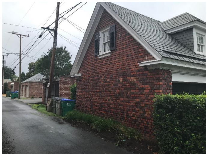
Figure 4. View west of the east wall where the new niche, fixed glazing, and curved wall are proposed.
