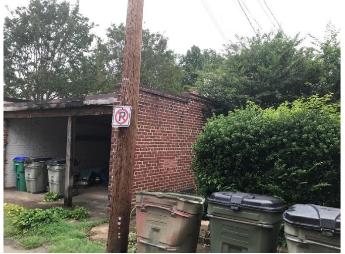
Figure 2. Existing east wall of the garage
