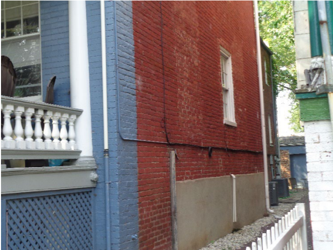
Figure 5. Number 412 West Marshall Street has a large, two-story, rear addition.
