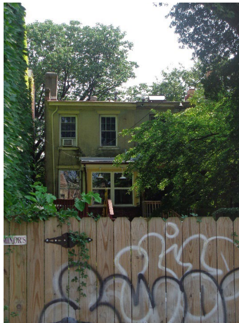
Figure 4. Zoomed in view of the rear of 414 West Marshall Street.
