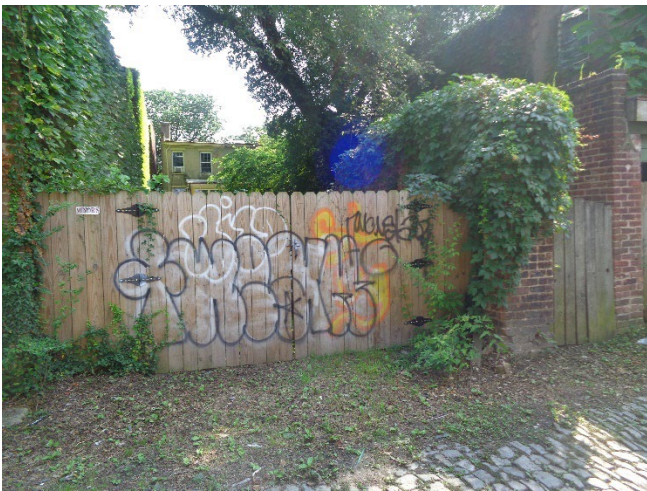
Figure 3. View of the rear of 414 West Marshall Street, from the alley.
