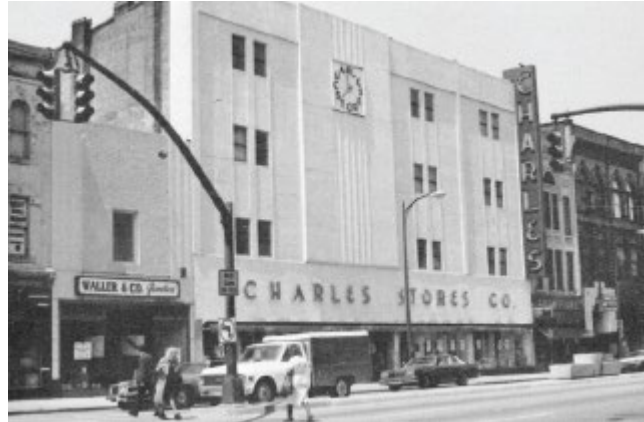
Figure 2. Original building after front façade alterations. Demolished 1989
