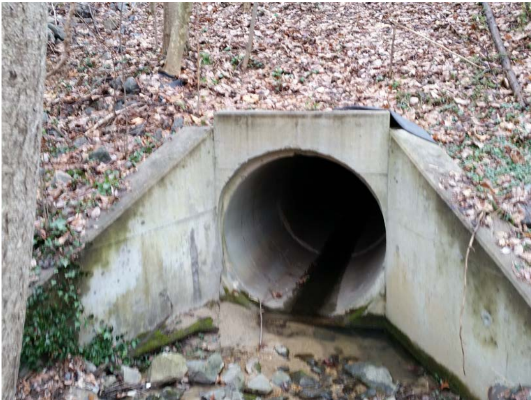
Upstream reach of perennial stream through 72" RCP on-site
