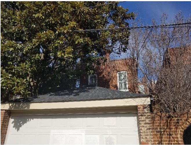
Figure 3. 2229 Monument Avenue, view off rear section roof.
