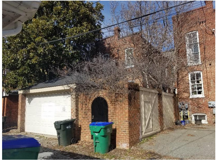
Figure 2. 2229 Monument Avenue, view towards to rear section roof.
