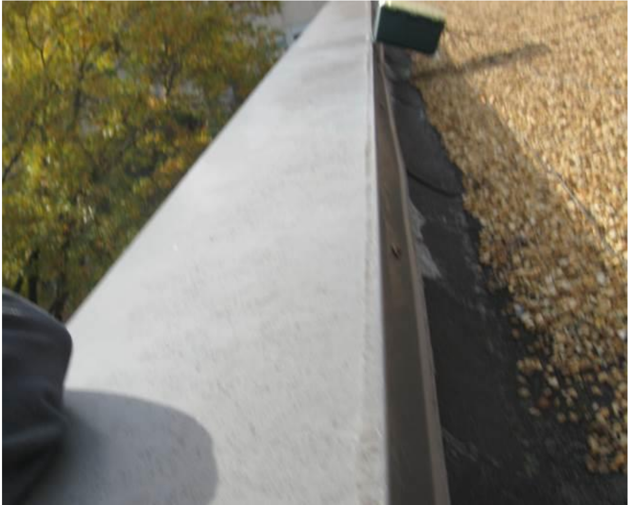
Figure 11: This image shows the roof flashing and gravel.
