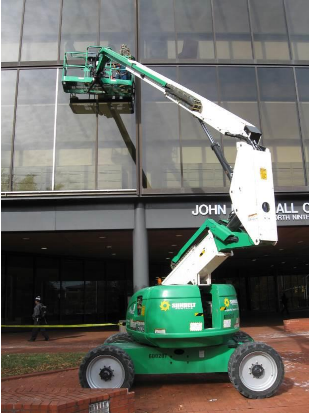
Figure 2: An articulating boom lift was used at the site.
