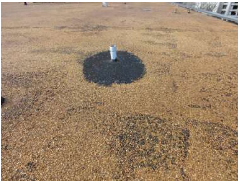
PATCH ON ROOF
