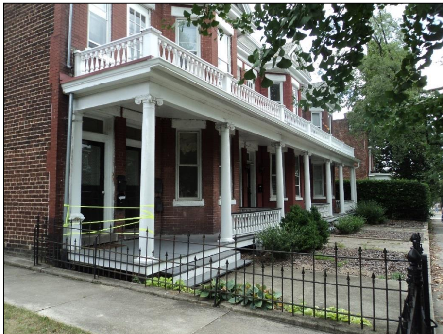
2708 - 2712 East Broad, New Gutters.
