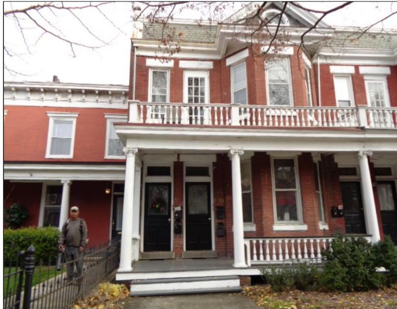
2708 East Broad Street, Assessor Photograph, date unknown.
