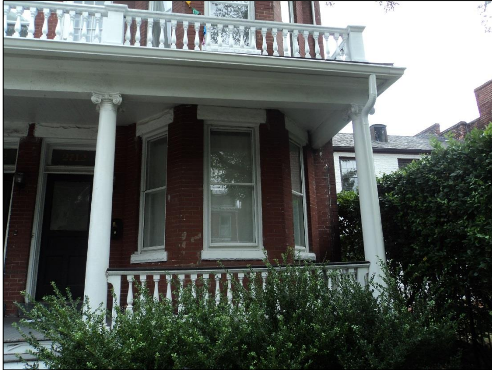
2712 East Broad Street, New Downspout.
