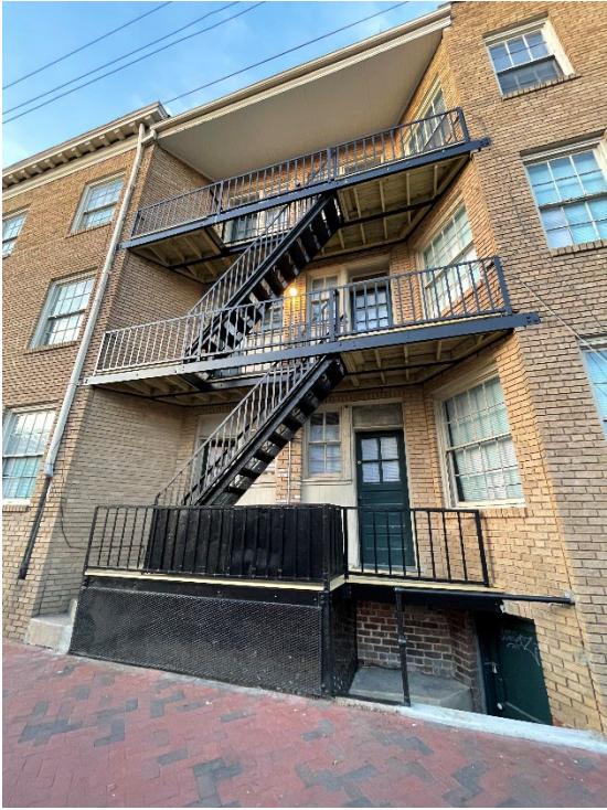
Figure 4. View of the fire escape on the south side of 23 South Arthur Ashe Boulevard. The new floor boards and their exposed decking can be seen on the second and third floors.
