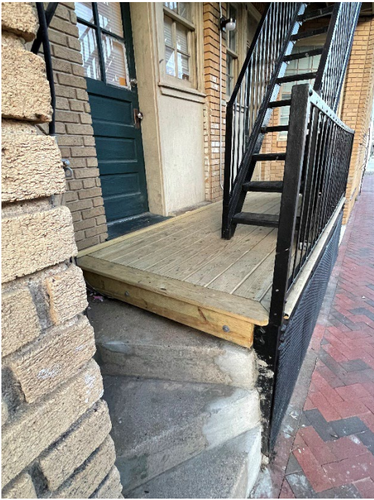
Figure 5. View of the replaced floorboards on the first floor of the fire escape on the south side of 23 South Arthur Ashe Boulevard.
