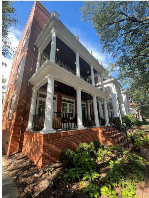
Figure 12. Photograph of 2901 Monument Avenue. This is a new construction, built in 2017, with fiberglass columns.
