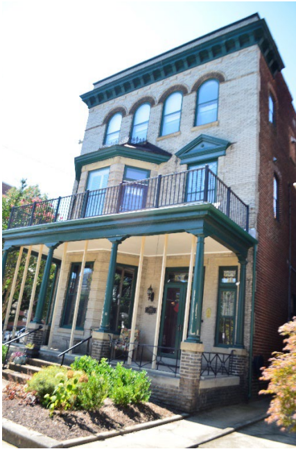
Figure 1. Façade of 2001 West Grace Street
