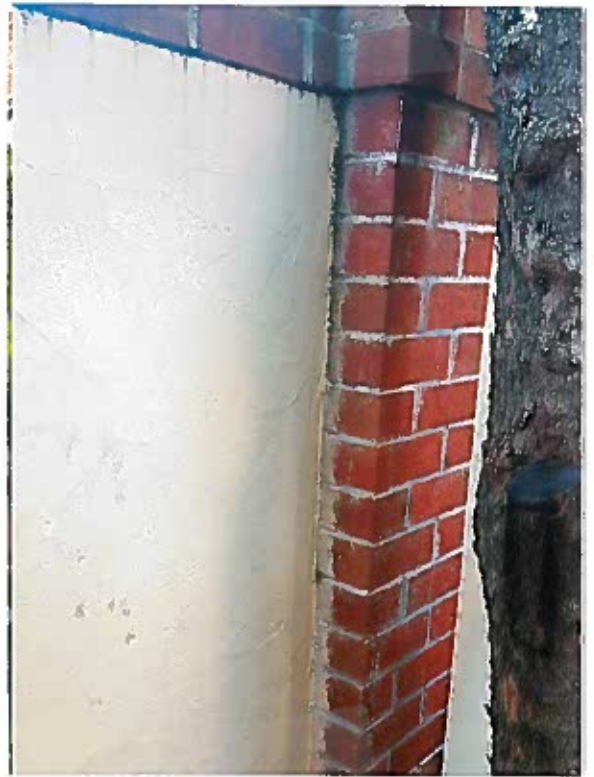
View of interior wall column
