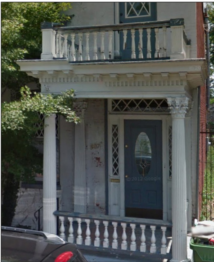
Prior to work performed (Google Streetview - July 2011)
