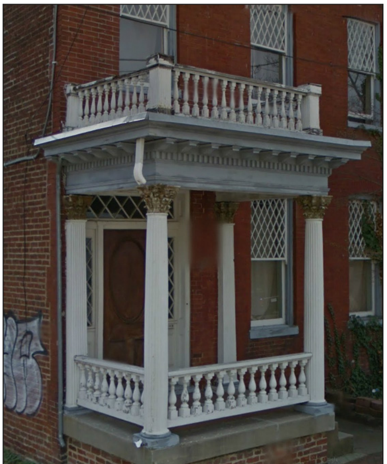
Existing balustrade at adjoining structure 509 N. Henry Street (Google Streetview - August 2014)
