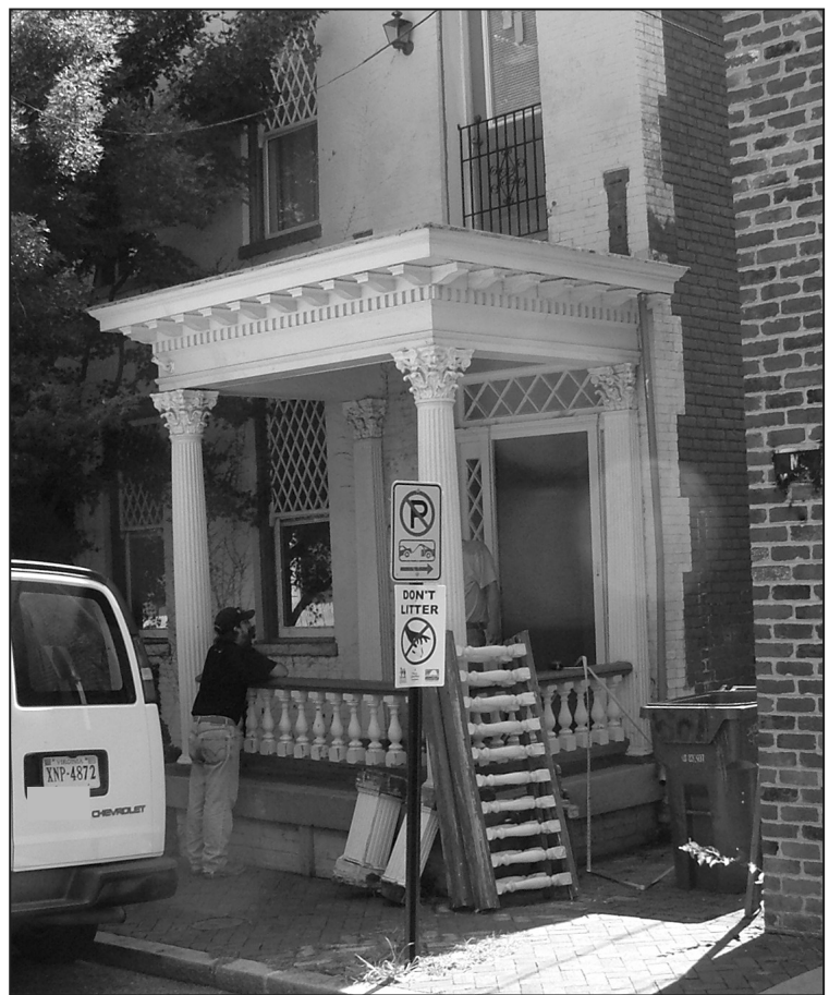
Work being performed (July 25, 2012)
