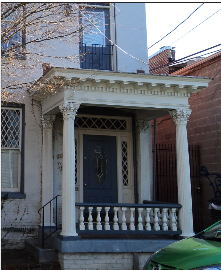
Current condition (January 5, 2015)
