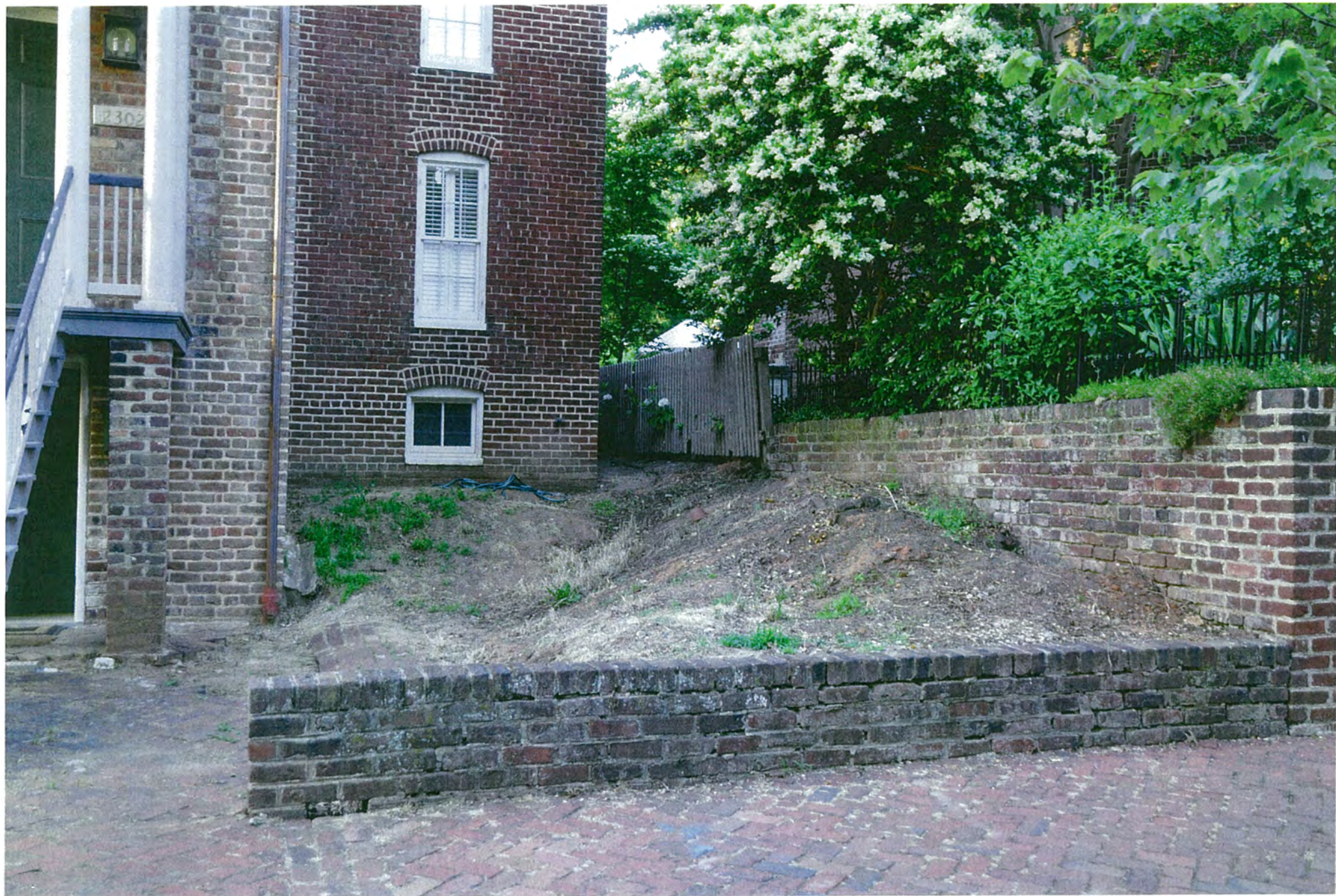
existing condition front east side
