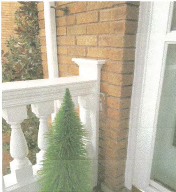
2 nd floor handrails
