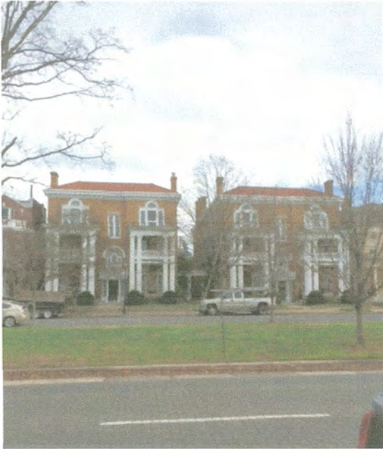
View from sidewalk across the street. Bottom of rails not visible.
