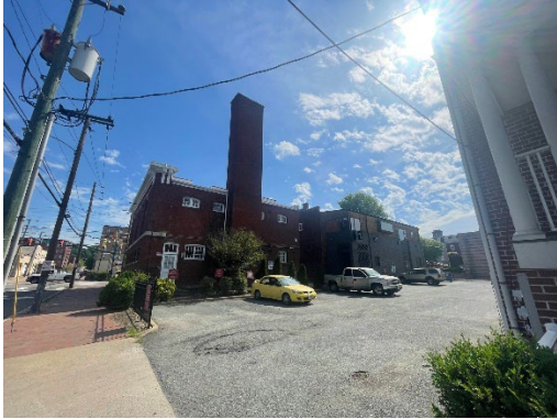
Figure 1. 1801 E. Broad Street. Chimney
