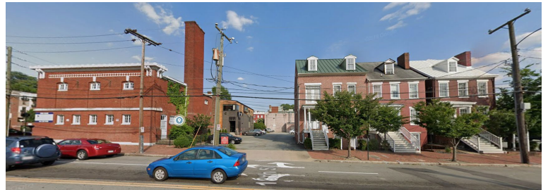
Figure 4. Site as seen from 18 th Street
