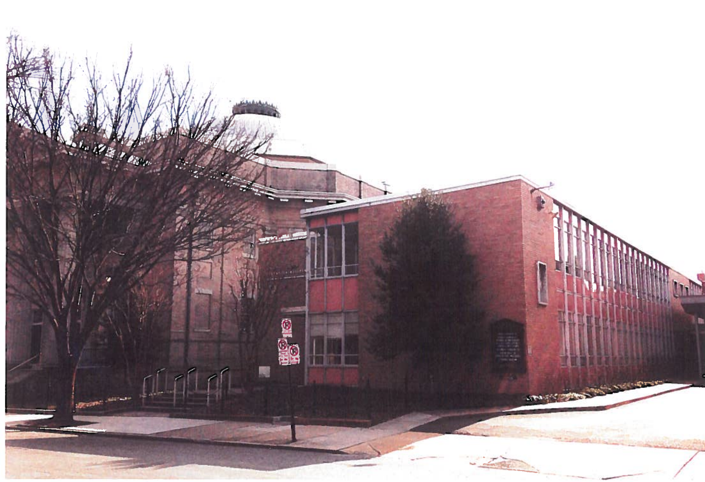
18| View of existing school facade from West Franklin St
