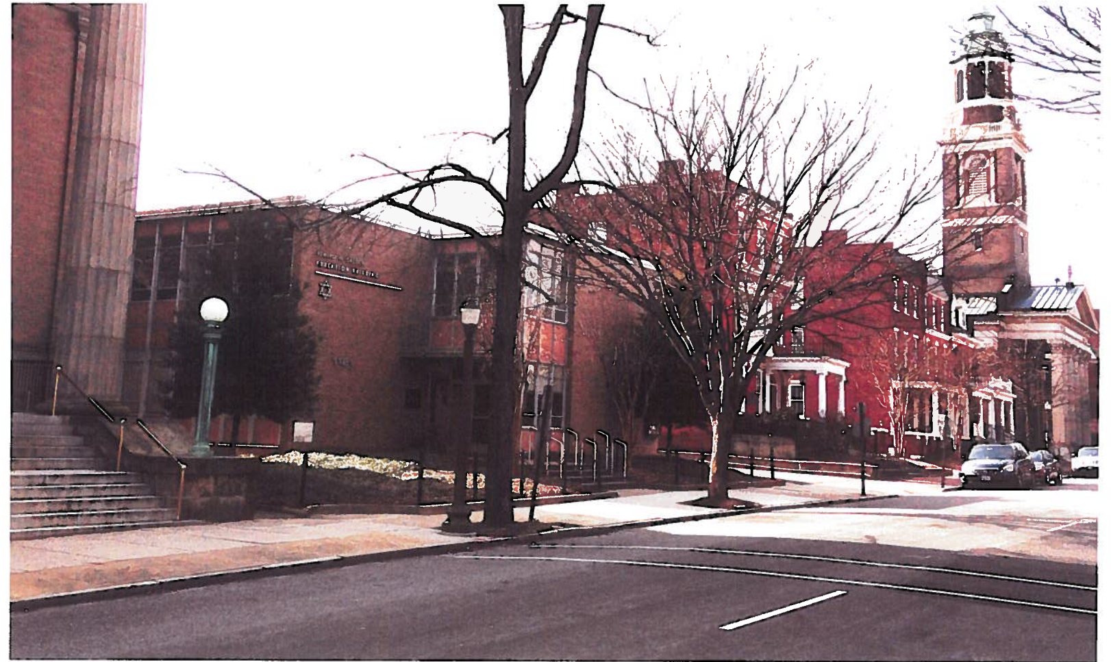
19| View of existing school facade from West Franklin St
