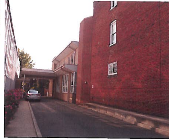
13| Link between 1121 and 1125, view of 1125 wall
