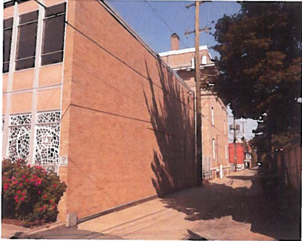
14| Alley view at back of 1121, toward 1117 Sanctuary
