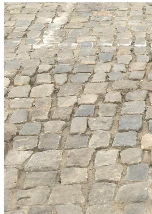
Cobble Paving Restoration
