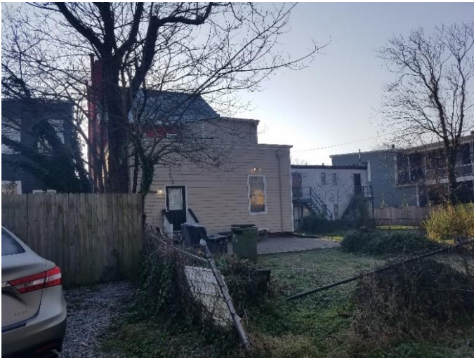
Figure 3. Rear massings on subject alley
