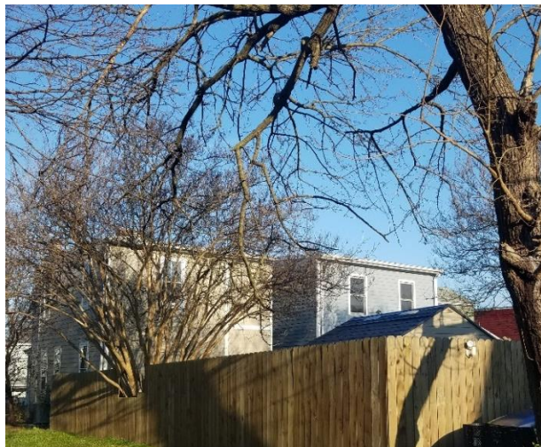
Figure 4. Rear massings on subject alley
