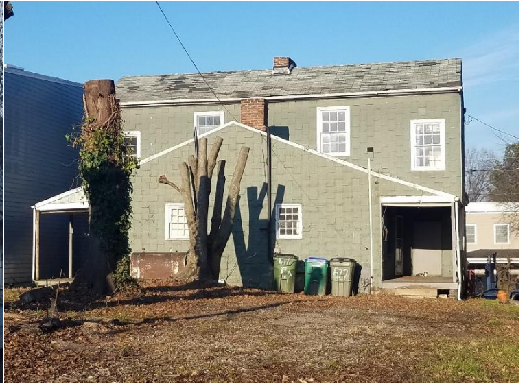
Figure 2. 515-517 North 28th Street, rear elevation
