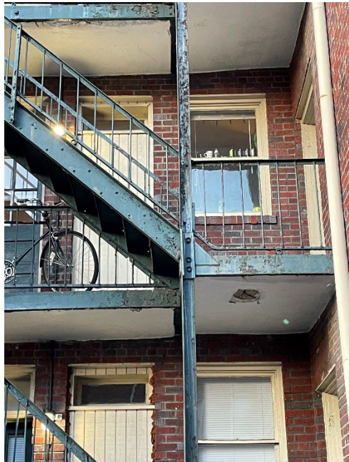
Figure 4. Zoomed-in image of deterioration of the steel and concrete floors along the second floor of the fire escape.
