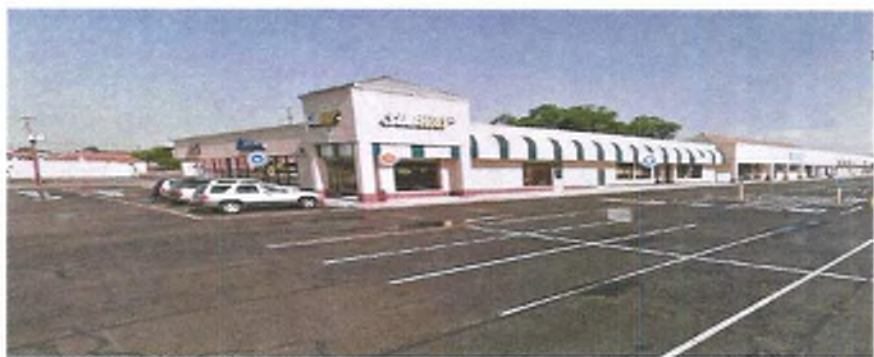
EXISTING SITE CONDITIONS
