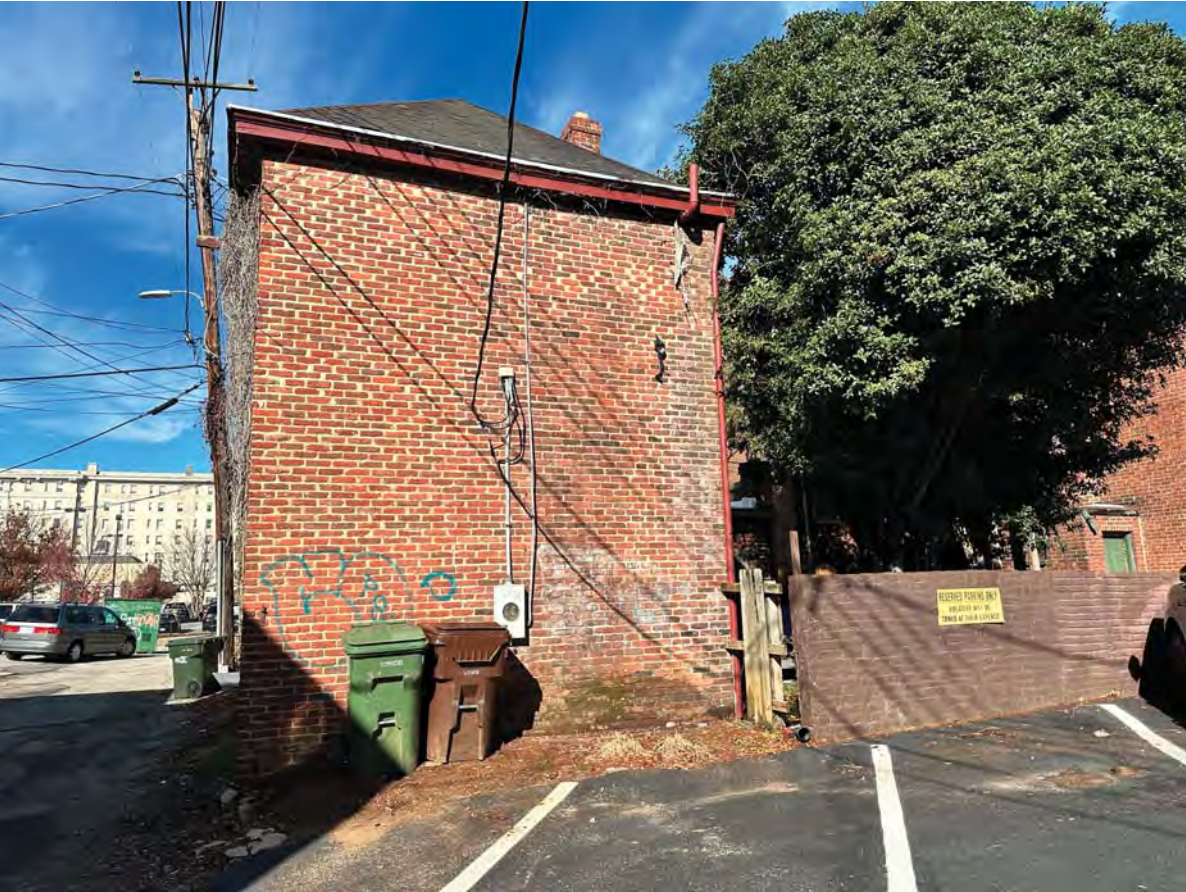
Carriage House – East & West Face
