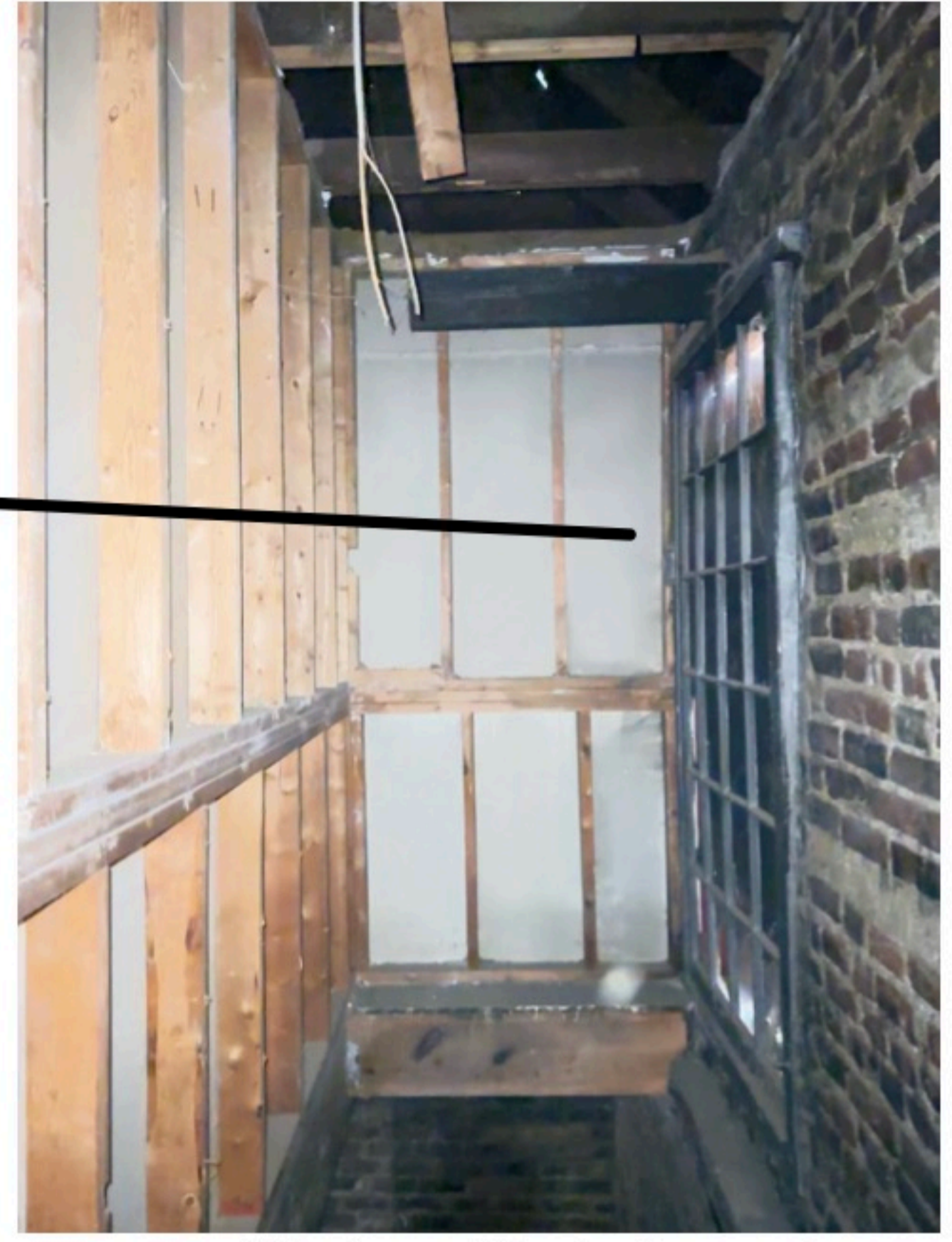
Window with glazing caving in, rear of building above staircase
