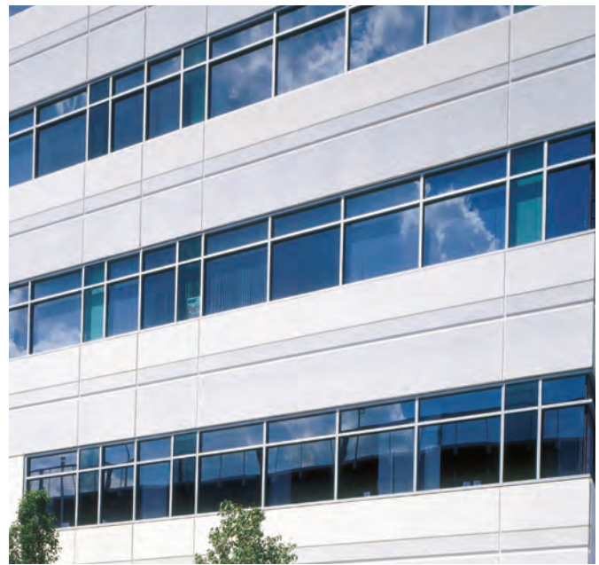
TSYS North Center, Columbus, GA Architect: C.S.I. Architects, Columbus, GA Glazing Contractor: Uneeda Glass Co., Columbus, GA
