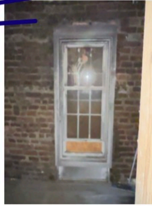
Front, center windows
